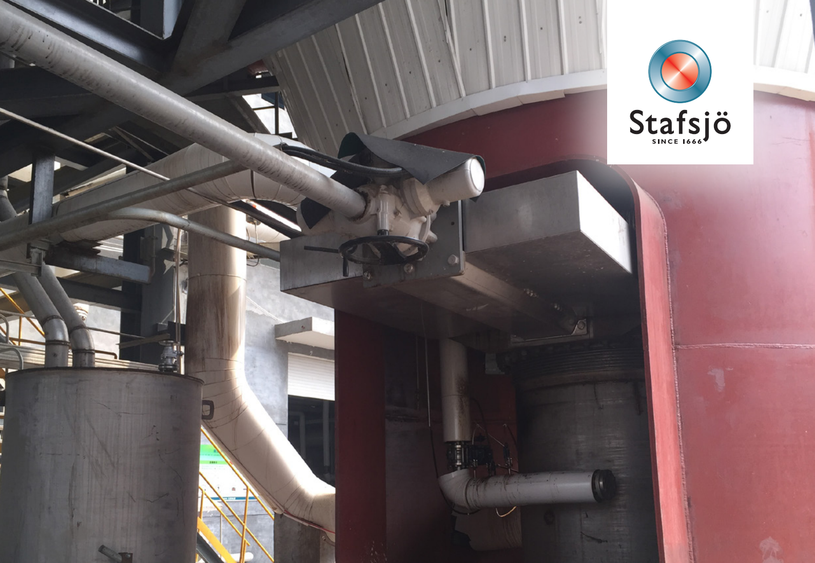
MV DN 1600 (64") installed on a gigant pulp and paper mill in China
